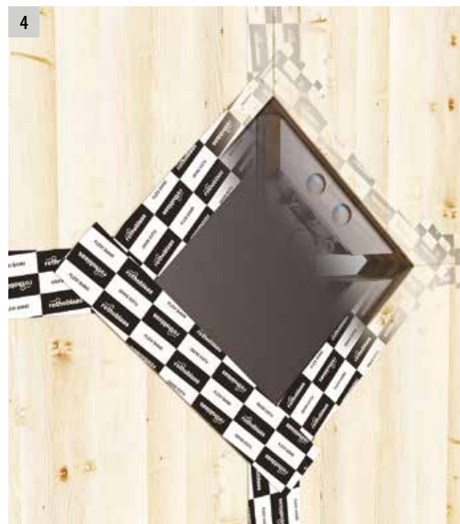
2. Attaching the wall to the ground 4. Sealing the connection
