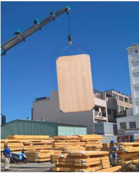
transporting the panels
