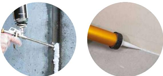
Sealing a through gap can produce an improvement of up to **+ 24 dB**.
