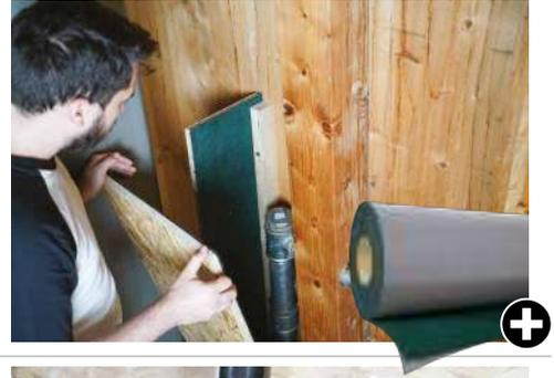
Seal any gaps created by the MEP penetrations with **HERMETIC FOAM** or **FIRE SEALING SILICONE**
