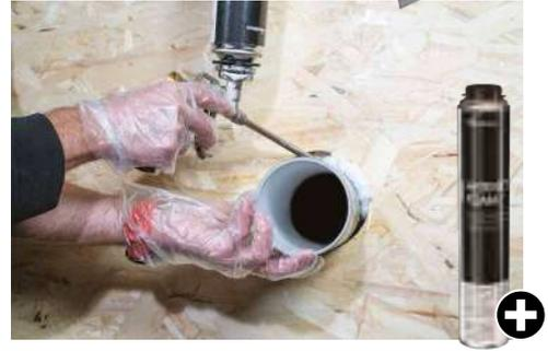
Place a resilient layer **PIANO A**, **SILENT FLOOR PUR** in strips, **SILENT FLOOR TEX** in strips, **SILENT UNDERFLOOR**, **GIPS BAND**, **CONSTRUCTION SEALING** between the MEP components and the fixing system to avoid rigid contact with other elements.
