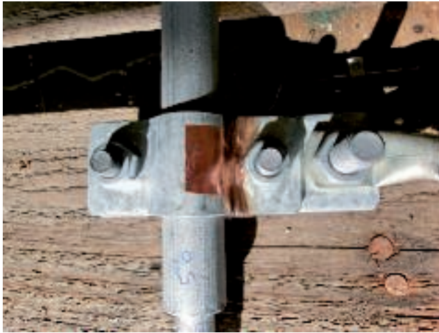
Short-circuit current test on earth rod terminal
