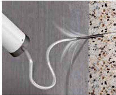
Cleaning of the drill hole Blowing out of the drill hole for cleaning with a hand-held blower or compressed air.
