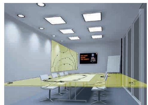
Approximately 450 lux is achieved at the user's eye. Optimum support of the biological system for middle-aged users.
