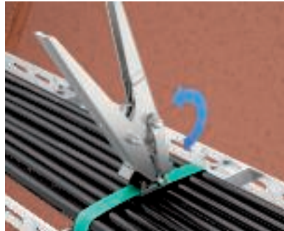
Shortening the tightening strap Turn the tightening strap over to prevent it from slipping out and shorten it as required (e.g. using metal cutters).
