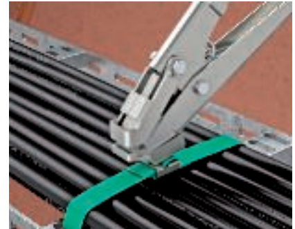
Knock the retaining strap over Using pliers, knock the retaining straps tight.
