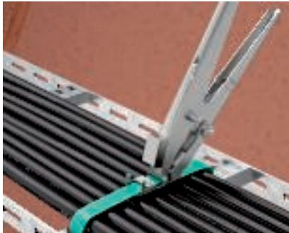
Tensioning Insert the end of the cut-out in the spring chuck, type 575 and tension it.
